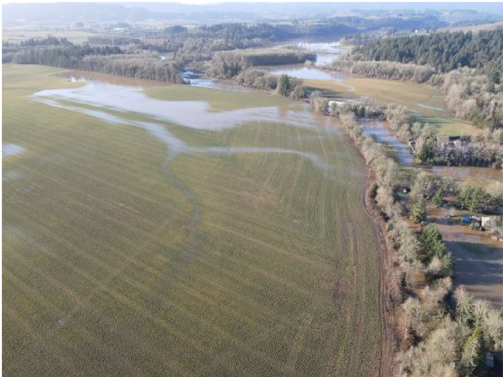
Drone Photo 14: View of W. Fork Dairy Creek and Straight Channel flooding into site on January 13, 2021, facing west.
