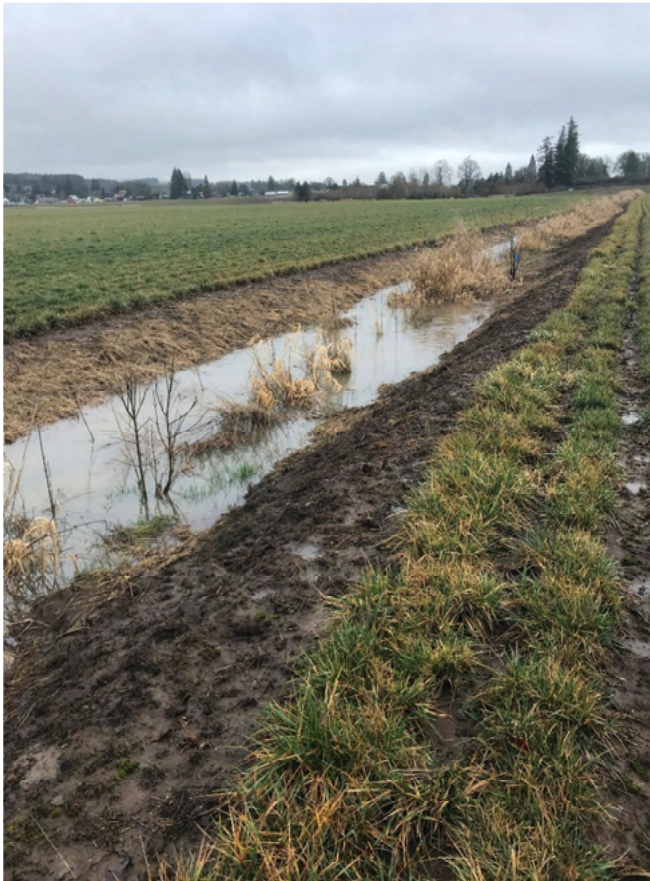
Photo 5: View of inundation in P2 East-West ditch on January 6, 2020, facing northeast.
