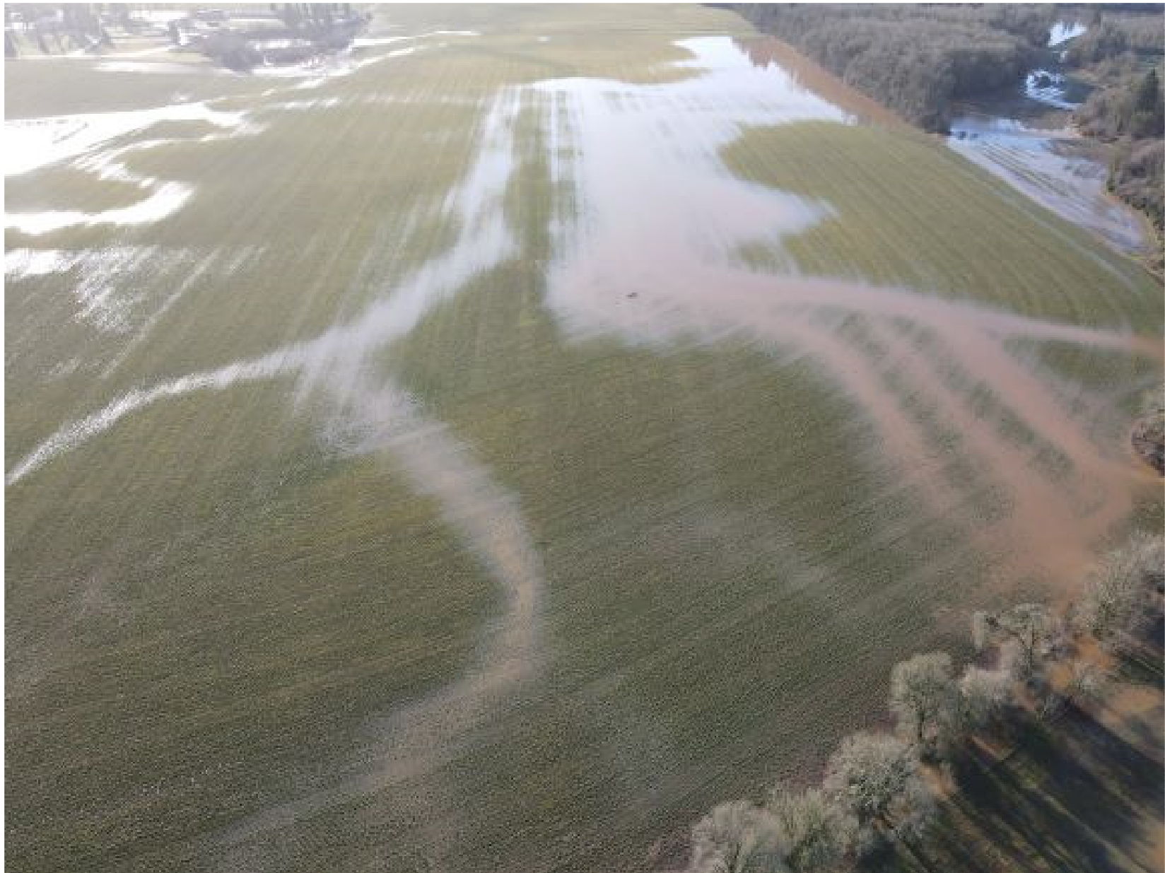
Drone Photo 16: View of flooding into DCMB from W. Fork Dairy Creek and Straight Channel in approximate location of proposed channels. Photo taken on January 13, 2021, facing south.
