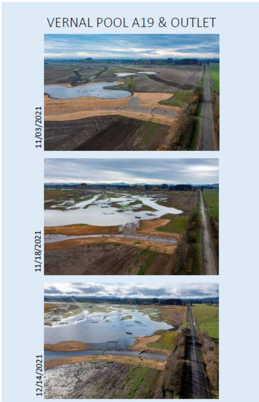
Figure 3.2. Drone photos of Pools 19 and 16 and the coir-covered north outlet over a 6-week period from early November to mid-December 2021.
