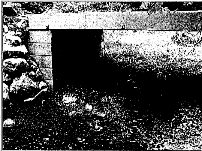
Photo # 2 West "Square Corner" Support Abutment Without Wingwalls Using Pacific Bridge "Mono" Abutment Units With "Returns"
