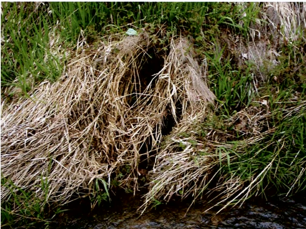
Photo 4. View looking west of creek outfall into right bank. Photo CMW 4/29/09
