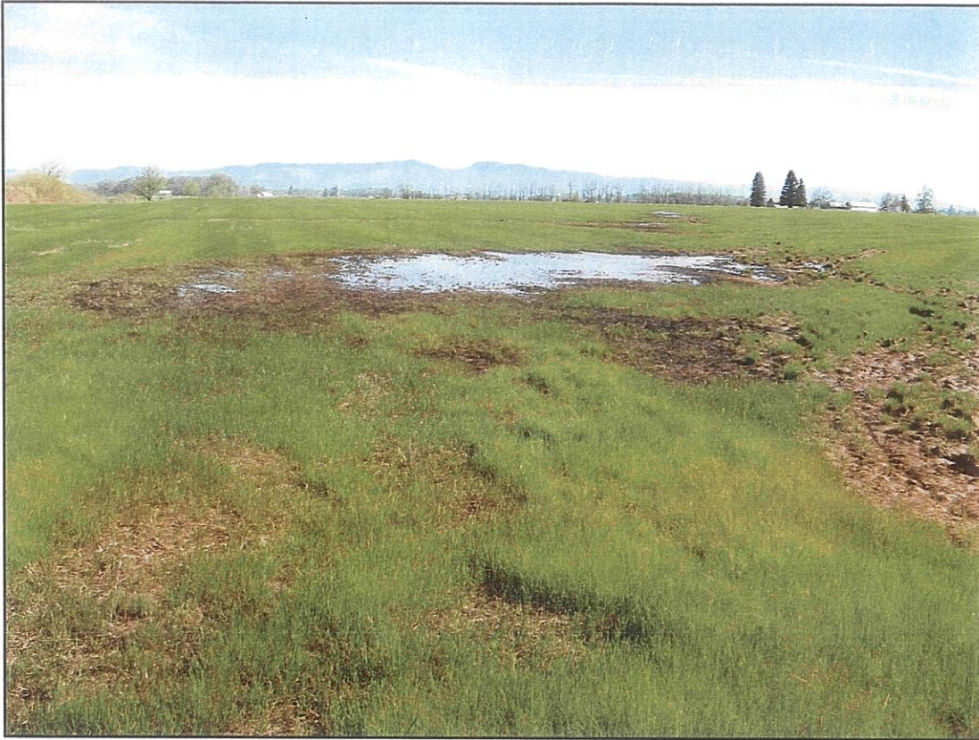
Photo 23: East field looking north on 3/16/07
