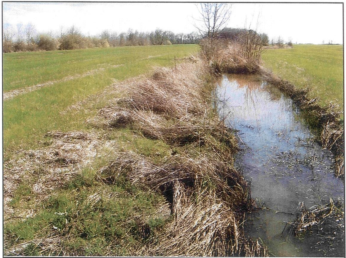
Photo 22: Drainage channel looking north on 3/16/07
