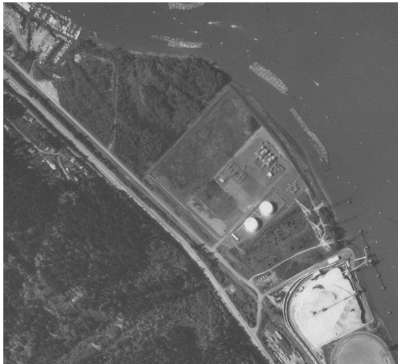
Photograph 4. 1980 aerial photo. Image depicts completed substation with generation and fuel storage facilities. Note formation of wetlands in undeveloped portion of the Property.
