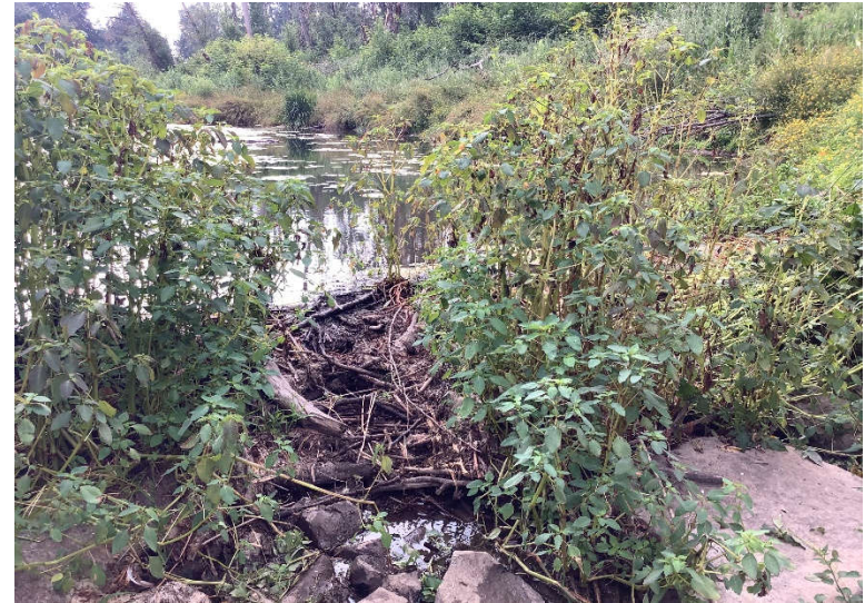
Figure D-6: Conditions at the pond outlet looking upstream, July.
