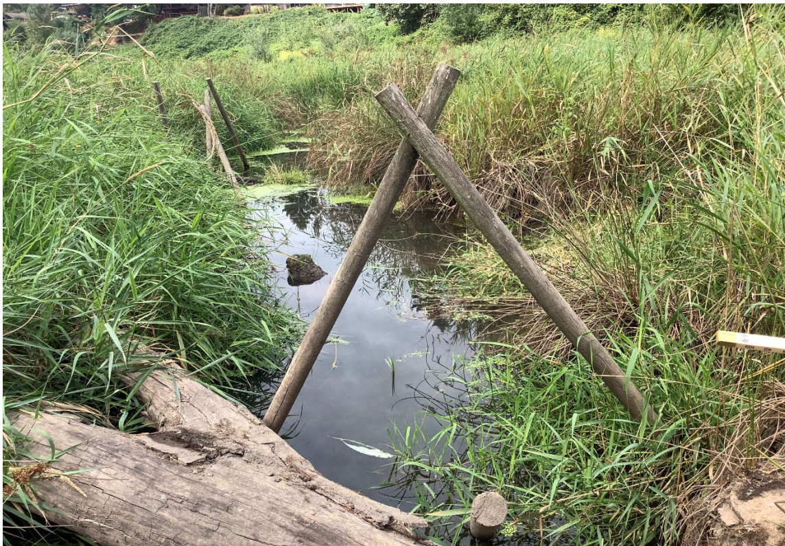
Figure 7-1. Floodplain channel section where head-cuts were previously reported but not found in Year 3 monitoring.
