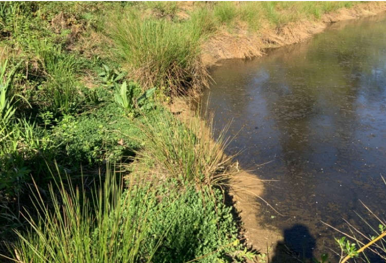
Figure D-3: Conditions at the pond outlet, May.
