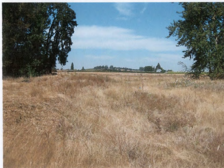
Photo Point 4 N: Photo displays the head of the constructed swale, at the un-improved access road crossing.
