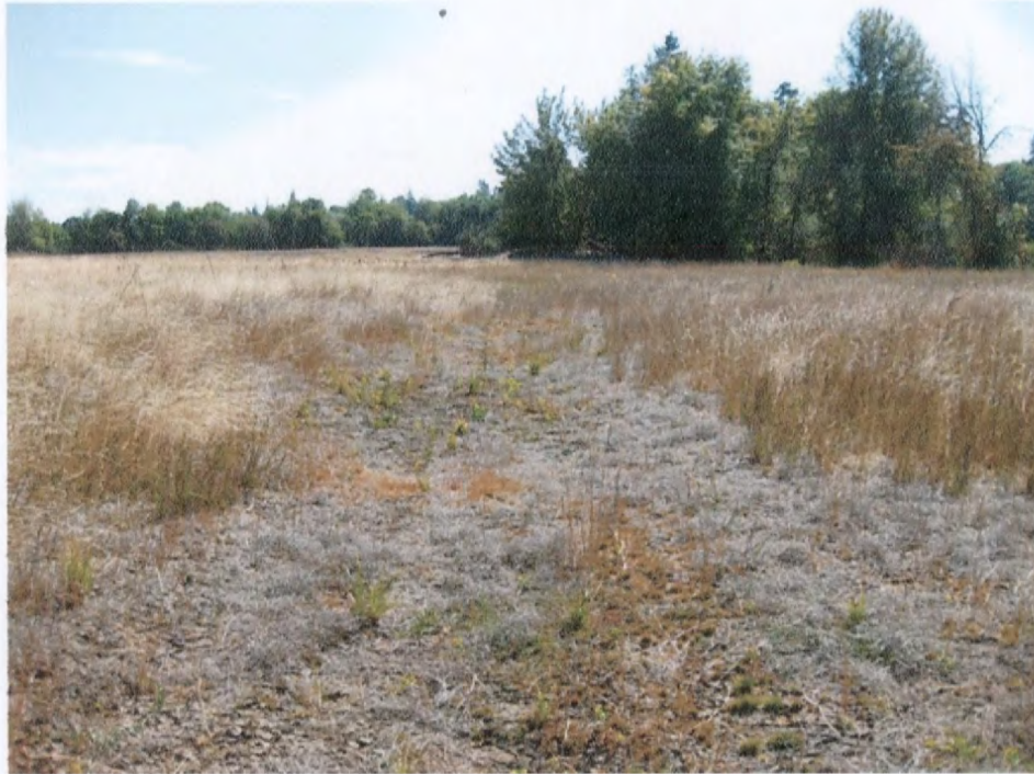
Photo Point 11 SE: Photo displays the mouth of the constructed swale looking toward the log jams.
