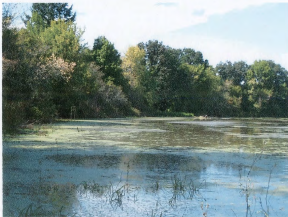
Photo Point 14 NW: Photo displays the re-contoured location of the 18” culvert and ditch outfall.
