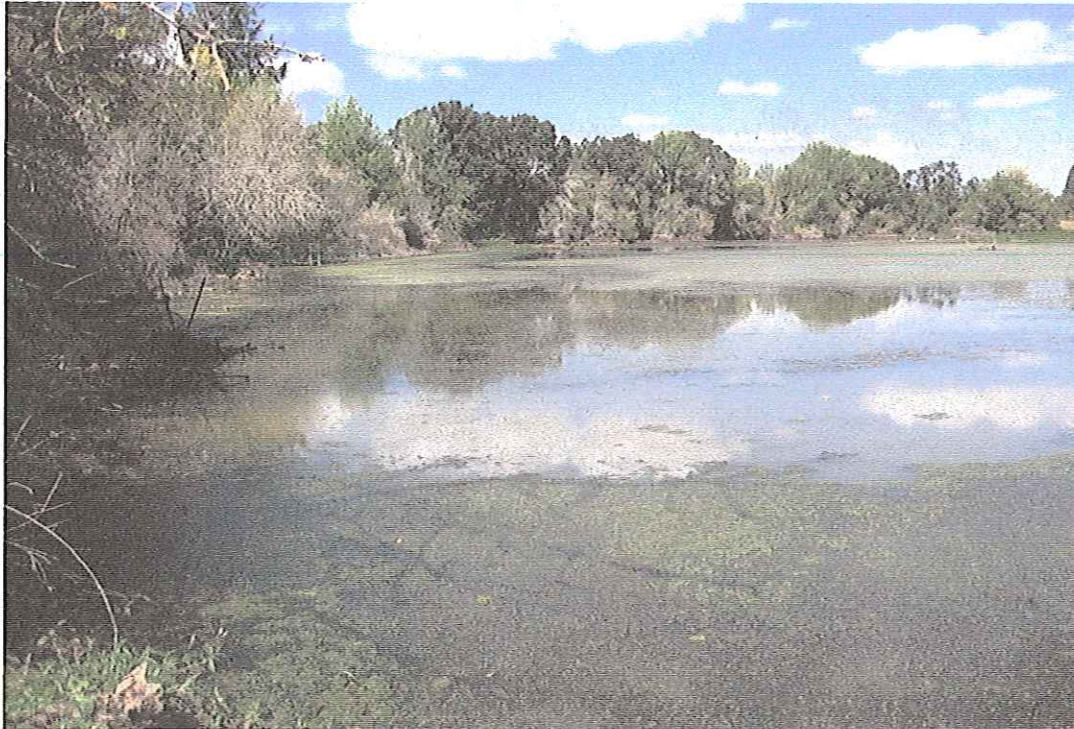
Photo Point 14 NW: Photo displays the re-contoured location of the 18" culvert and ditch outfall.
