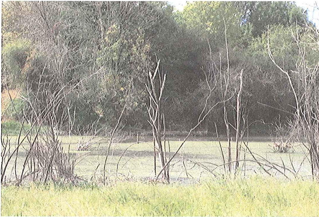
Photo Point 13 SW: Photo displays the re-contoured location of the 18" culvert, ditch outfall, and adjacent hill-slope trench.
