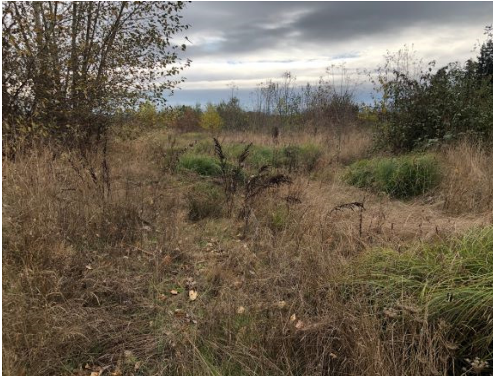
Photo Point 4 S: Photo displays head of constructed swale, at the un-improved access road crossing.
