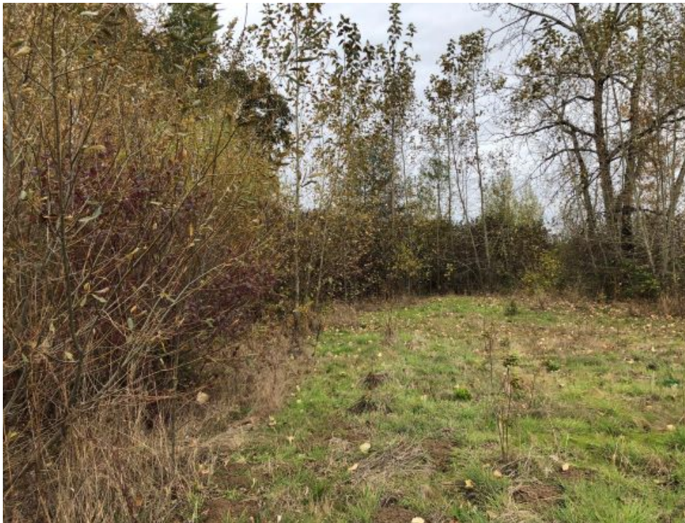
Photo Point 4 N: Photo displays the head of the constructed swale, at the un-improved access road crossing.
