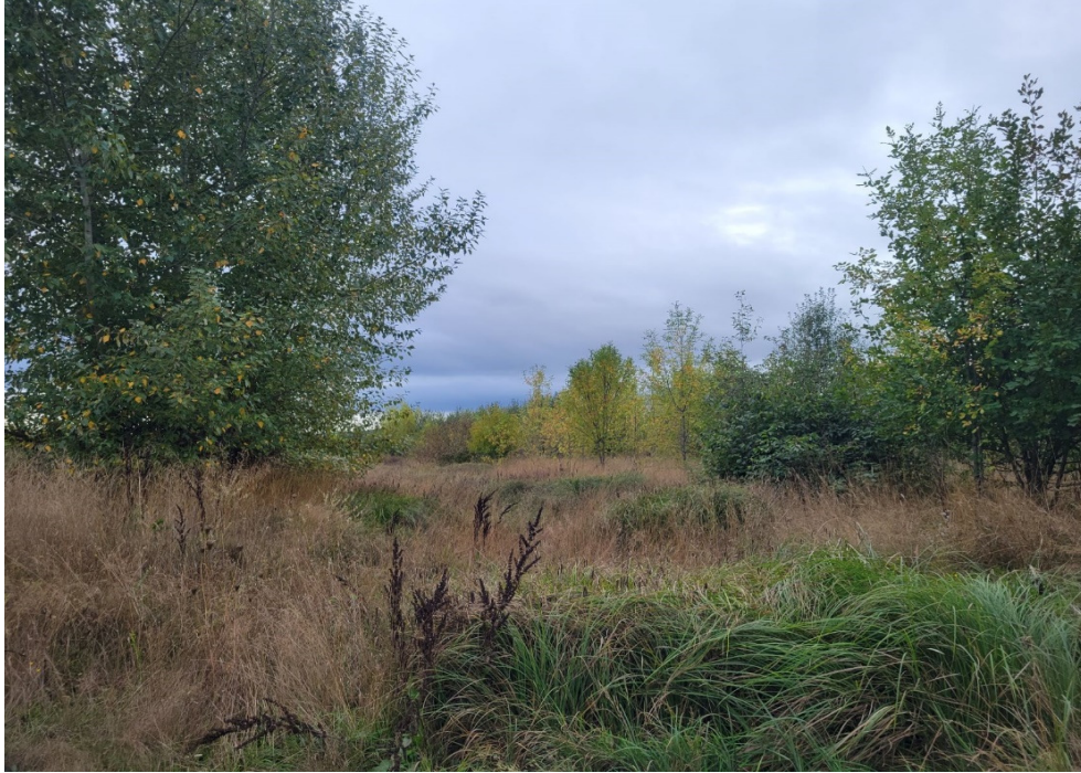
Photo Point 4 S: Photo displays head of constructed swale, at the un-improved access road crossing.
