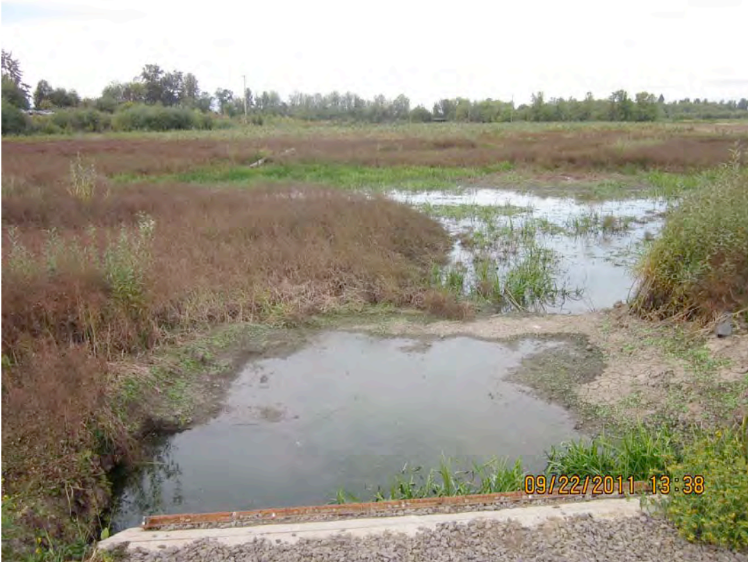
Photo 3 - Access road intersection facing northwest overlooking culvert inlet from new slough.
