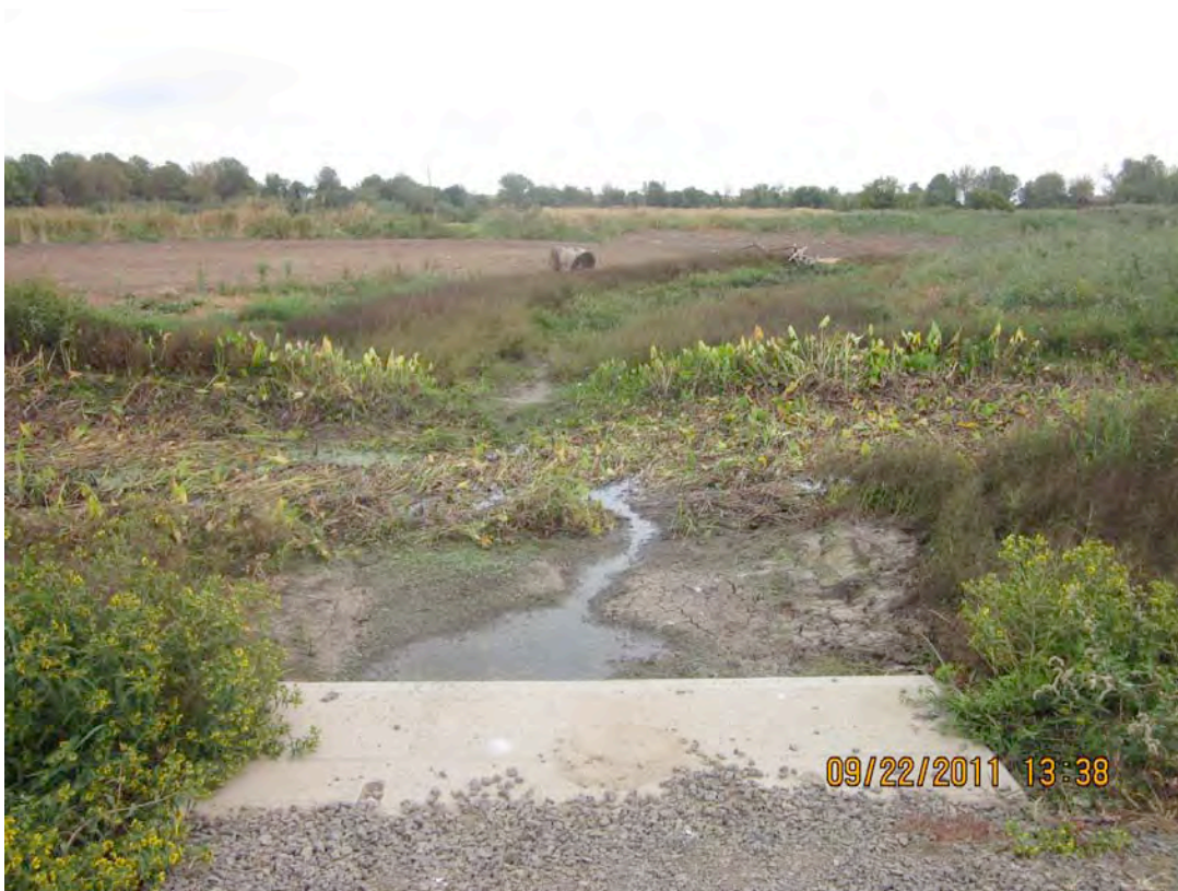
Photo 2 - Access road facing southeast overlooking culvert outlet to new slough channel.
