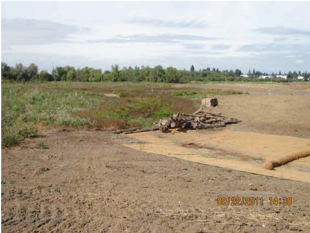
Photo 24 - East outlet slough facing northwest.
