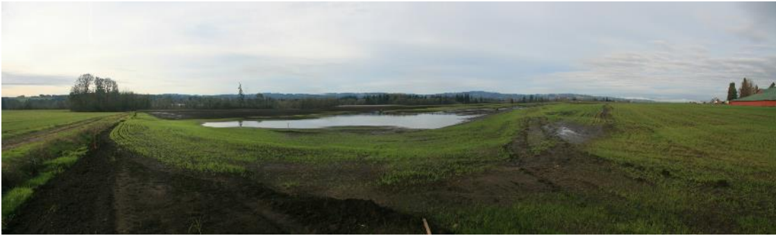
11/2014- After initial phase of construction and before planting.
