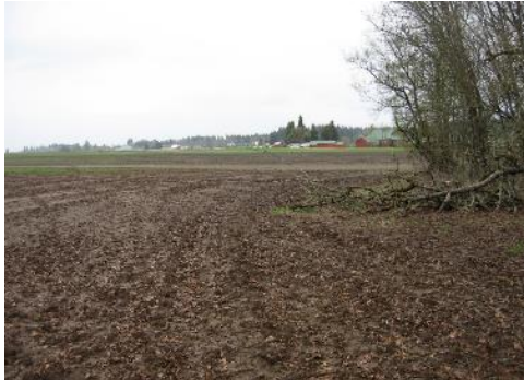
3/2014- During site prep phase for east field
