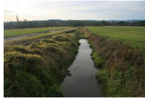
11/2014- After initial phase of construction
