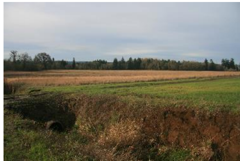
11/2014- After initial phase of construction
