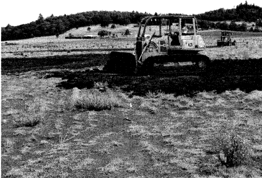
Figure 2. Coyote Prairie, East Phase, vernal pool excavation, summer 2009.
