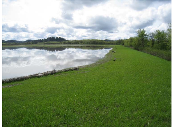
Fig. 2. From the water control structure looking south along west boundary berm. Northwest corner still has several inches of water when photo taken April 15, 2016.
