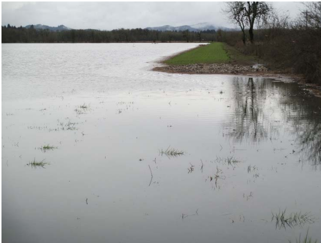
Fig. 1. Dec 18 2015 water levels in northwest corner of West Phase. Photo taken near parking pad looking west at berm's east end.
