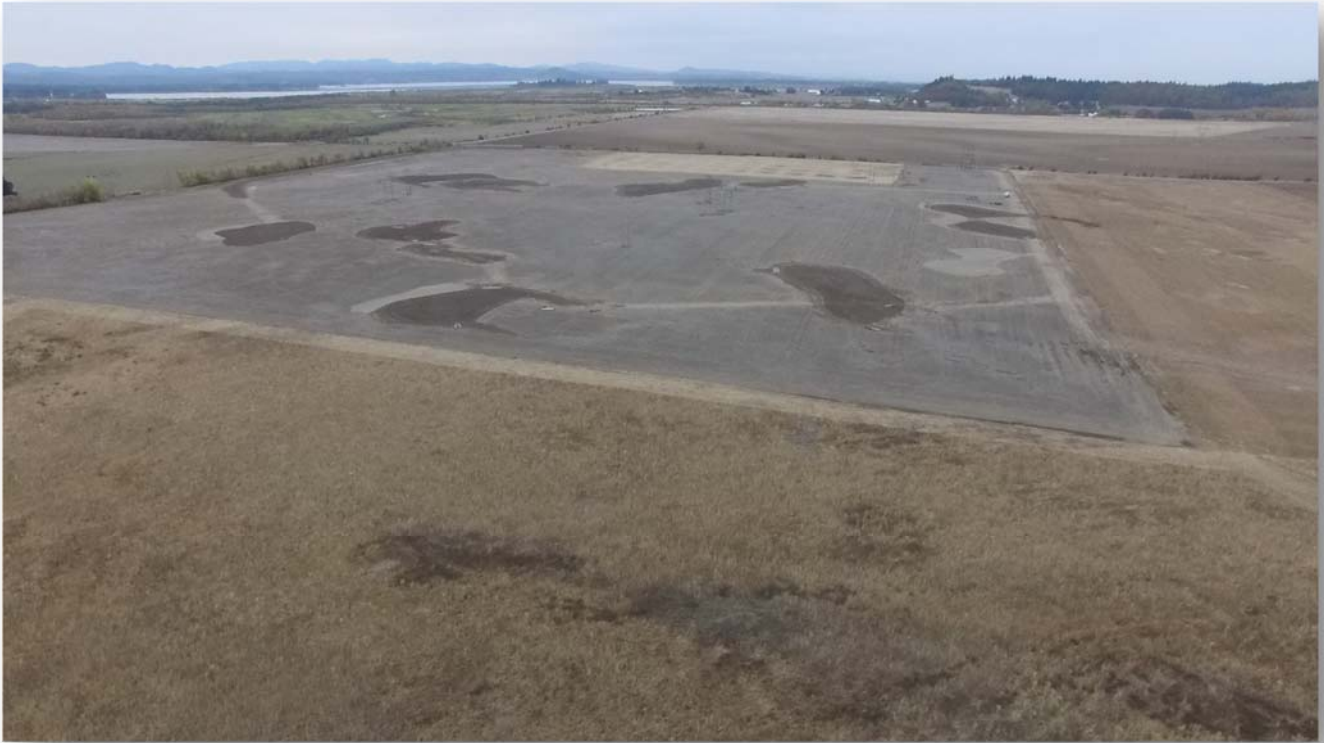
Aerial image of the West Phase and newly constructed vernal pools, taken October 16, 2015
