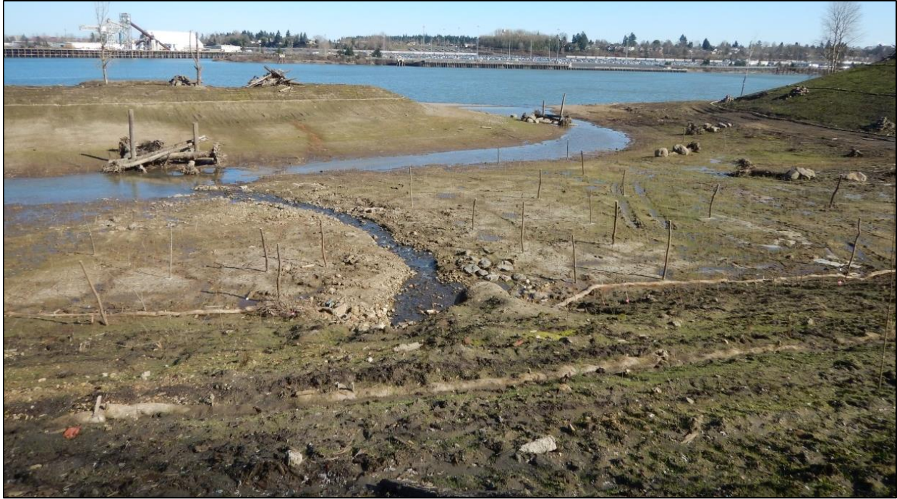
Photograph 12. Linnton Creek discharging 2/19/20, daylighting groundwater to the right, from Photo Point 12.
