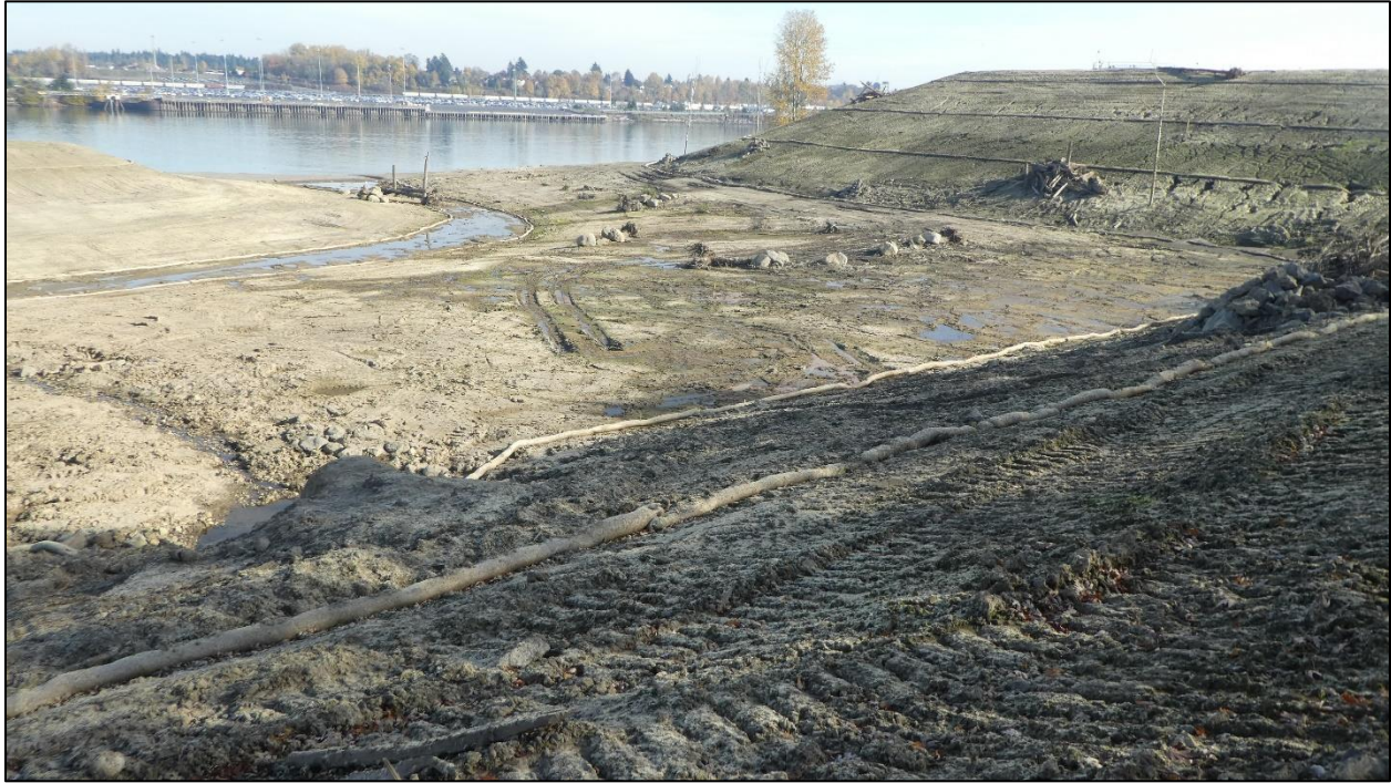
Photograph 9. Groundwater daylighting from the hillside, from Photo Point 12 11/9/19.
