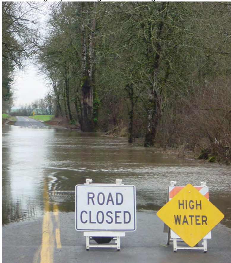
Flooded road, Willamette Valley
